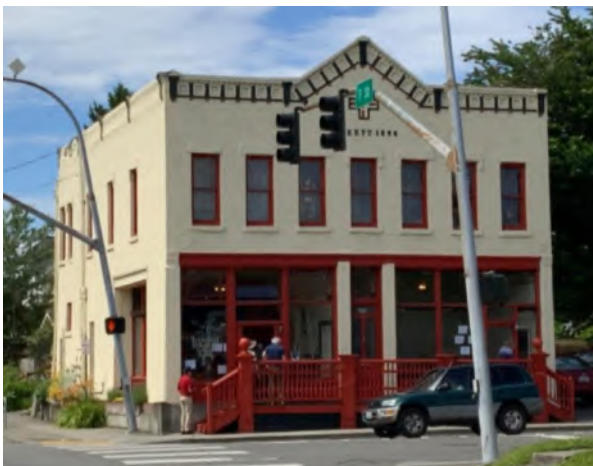
Figure 10. Oblique view of the building showing the Dupont and F Street facades.
