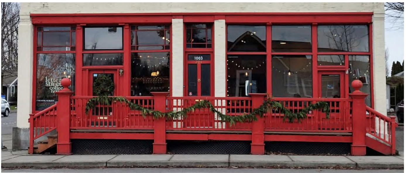
Figure 12. The main façade has a symmetrical layout to the commercial spaces, flanking the centrally located stairway door. It appears that three divided light transom windows remain intact, two on the eastern space and one over the upper story door. The western commercial windows are not symmetrical, suggesting that the entry door may have originally been located within the center window opening.
