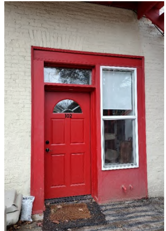
Figure 19. Note the vertical brickwork over the entry door to Apartment 102 under the stairway on the southwestern face, revealing the expansion of the opening to include a window next to the door.
