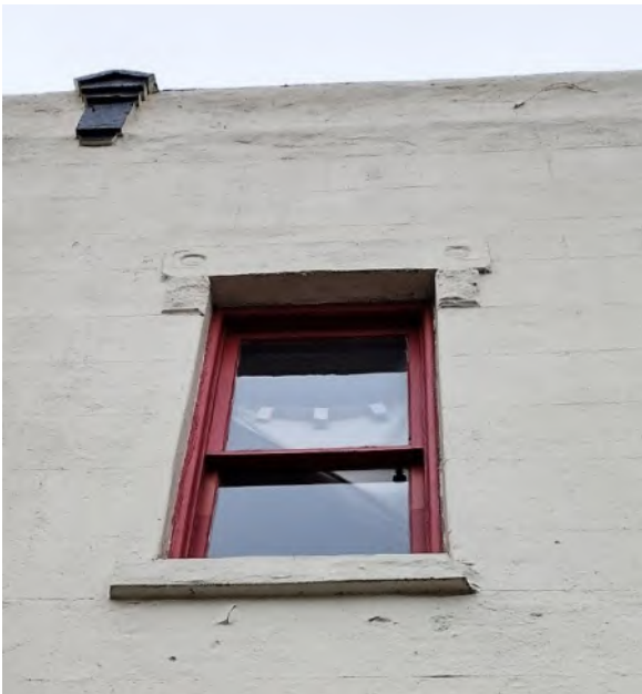
Figure 14. The F Street façade has had stucco applied over the brick and a faint faux block pattern traced into the stucco. Some of the original detail of the lintel, the lintel bracket, and the decorative bullseye remain.
