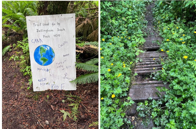
Figure 9: Volunteers have taken on some trail maintenance. Bridge shown on right needs repair.
