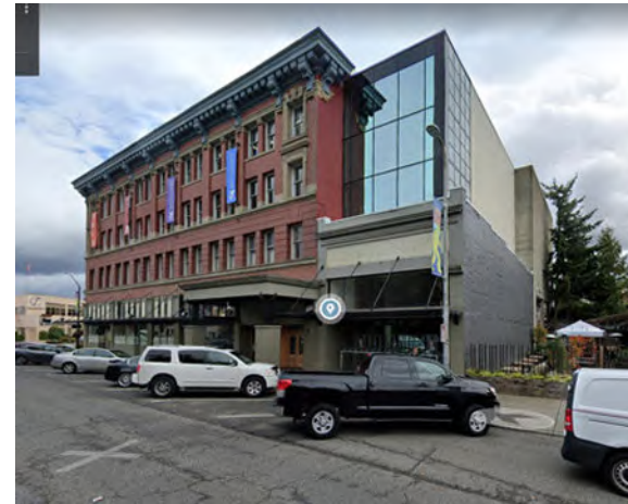
Set-back roof addition to historic commercial building
