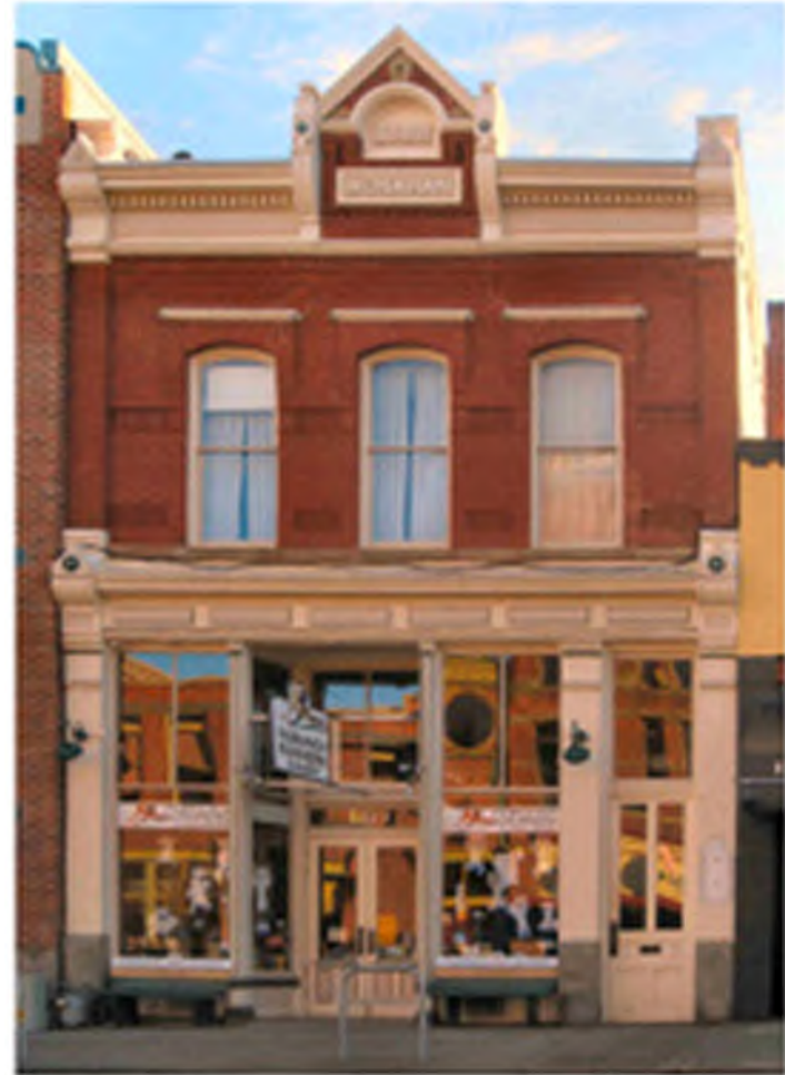
The Monahan Building in Fairhaven Historic District
