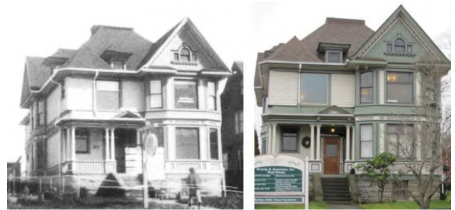
Many 20th century homes contribute to Downtown National Historic District
