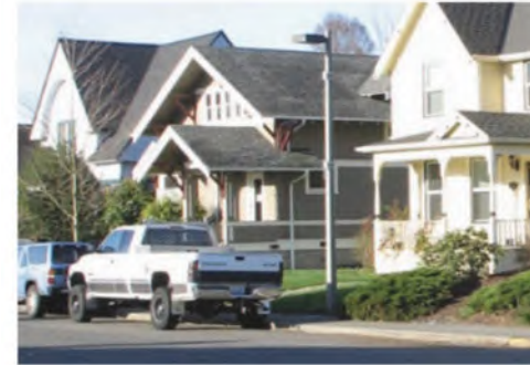
Historic homes turned offices in Eldridge National Historic District
