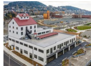
The Granary Building, Waterfront Urban Village .
