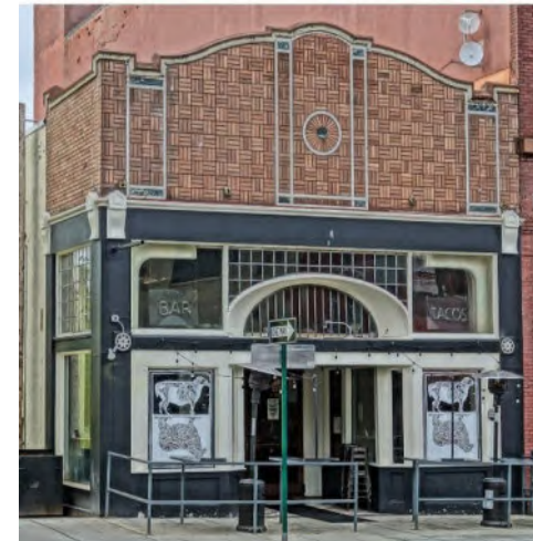
The Barlow Building, restored to original 1892 façade after past modernization effort
