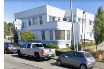
The Fountain Animal Hospital, built in 1940 in the Fountain District Urban Village , was designed in the Art Moderne style.
