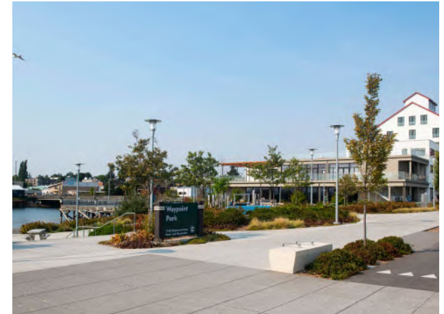
Granary Ave entrance to Waypoint Park with the Granary Building (1211 Granary Ave) to the right.
