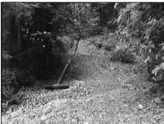
Wintercress Way Culvert Project Sudden Valley 2013
