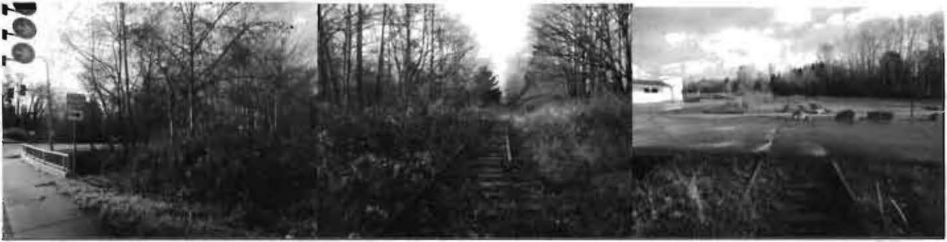
The Northern end of the line at the junction of Squalicum Parkway and Guide Meridian
